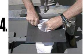
Place the snap band groove into the cell plate setting the seam of the bag first.
